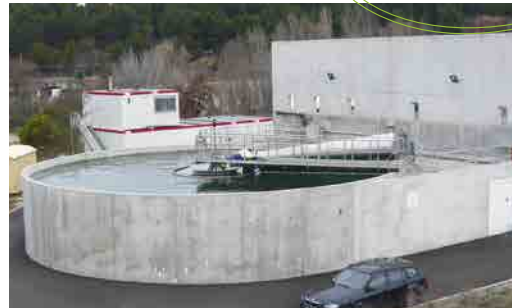
Municipal wastewater treatment plants Sludge thickening
